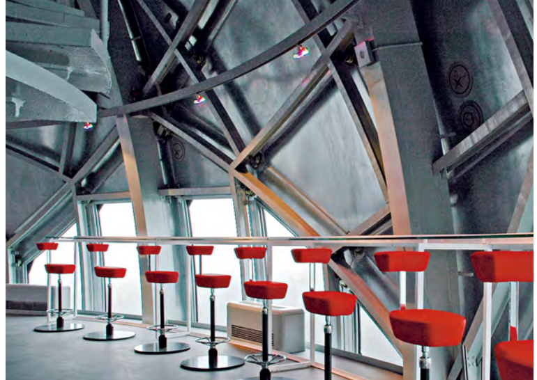
Inside the Atomium, the architectural design also supports the theme of scientific and technological advancement. The loadbearing frame and cladding panels are fully exposed.
