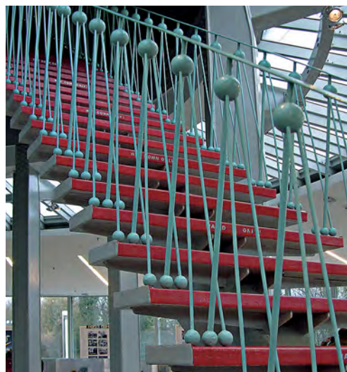
The original 1950s staircases and railings featuring 'atomic' sphere motifs were kept, and painted in red and pale turquoise.
