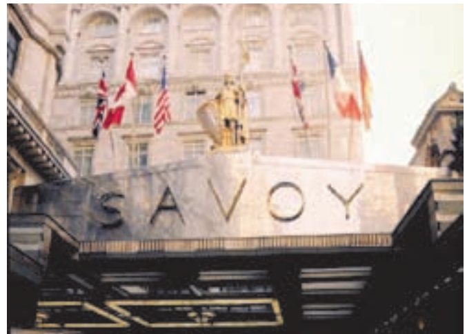
In 1999 the 70-year old entrance canopy at London's Savoy Hotel was cleaned, repaired and re-installed after the fire at the Savoy Theatre alongside (Courtesy of Outokumpu Stainless)
