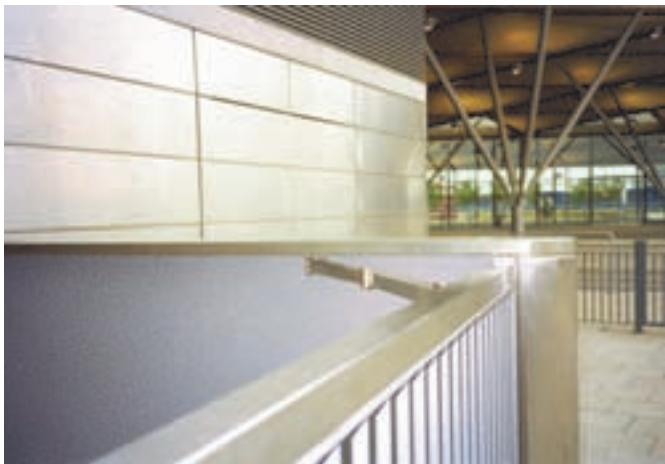
North Greenwich Underground Station: stainless steel combines modern design and durability in areas of high density use (Courtesy of Euro Inox)
