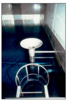
In the building of tanks for drinking water there are two very important aspects: perfect water tightness and hygiene. For the first aspect in general, waterproof plaster or impermeable cement mortar is used as covering. the high roughness of the surfaces and the imperfect planarity which creates areas of accumulation.
