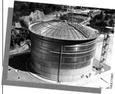
Matsuyama's municipal water tank is constructed of three grades of stainless steel: S30400, S31600, and S31803.
