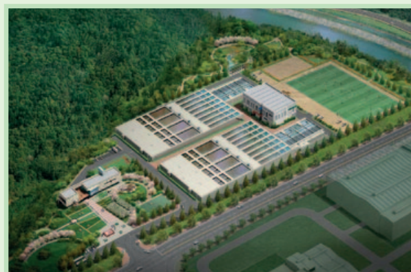
An example of a sewage plant, Paju, Korea. (Photo: POSCO E & C, Korea)
