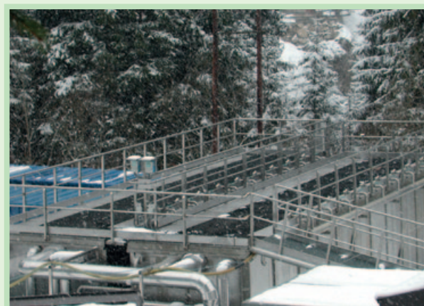
An entirely transportable stainless steel prefabricated depurator of San Martino di Castrozza, Italy (Photo: Centro Inox, Italy)
