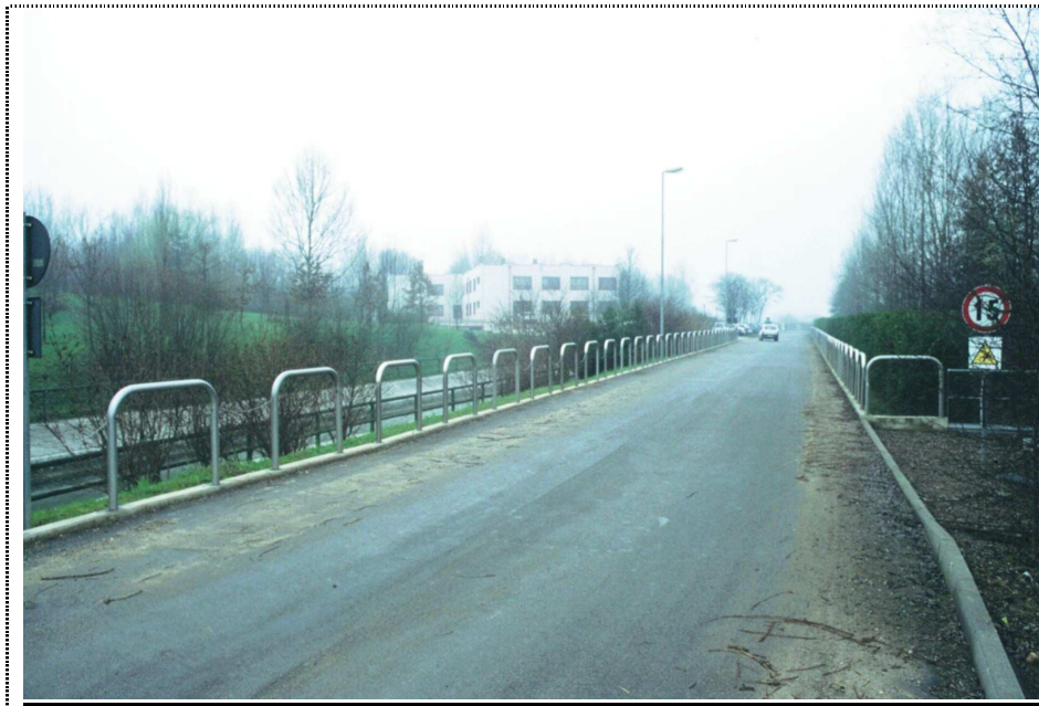
Figure 12. (March 2001). On the driveway connecting plant with the building office in the background, stainless steel arches and chains are installed to prevent car parking.
