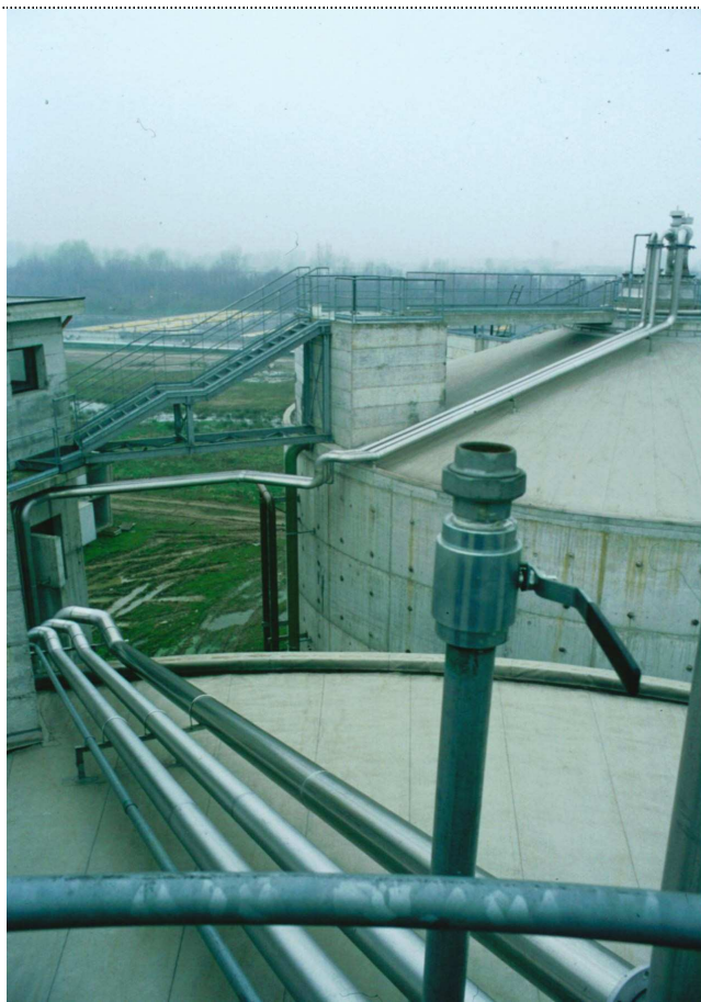
Figure 10. (March 2001) – Type 316 work pipe at the digester domes.
