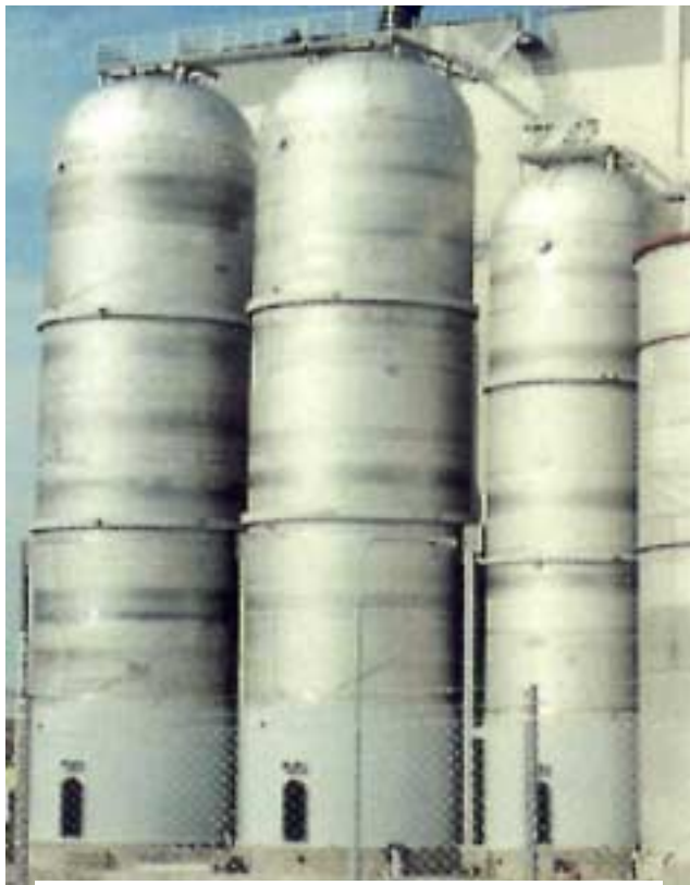
Fig. 3- UNS 32 304 and 31 803 Kraft Liquor Tanks (by courtesy of SUNDS DEFIBRATOR, Finland).
