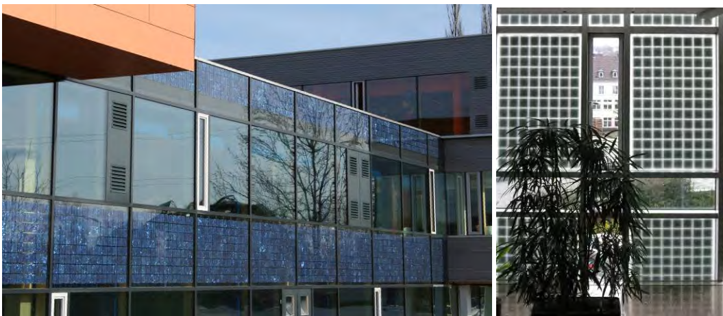
Fig. 31: Crystalline photovoltaic balustrade elements (left, Ertex Solar) and crystalline photovoltaic façade elements in metal framework, inside (right, STAWAG).
