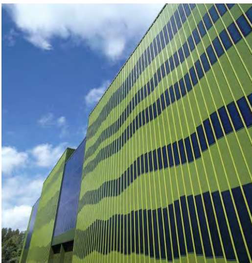
Fig. 31: Crystalline photovoltaic balustrade elements (left, Ertex Solar) and crystalline photovoltaic façade elements in metal framework, inside (right, STAWAG).
