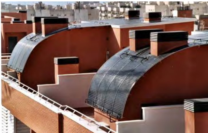
Fig. 23: Building-integrated low-temperature stainless steel thermal absorber in façades (top, Frei) and in roofs (bottom, Energie Solaire).
