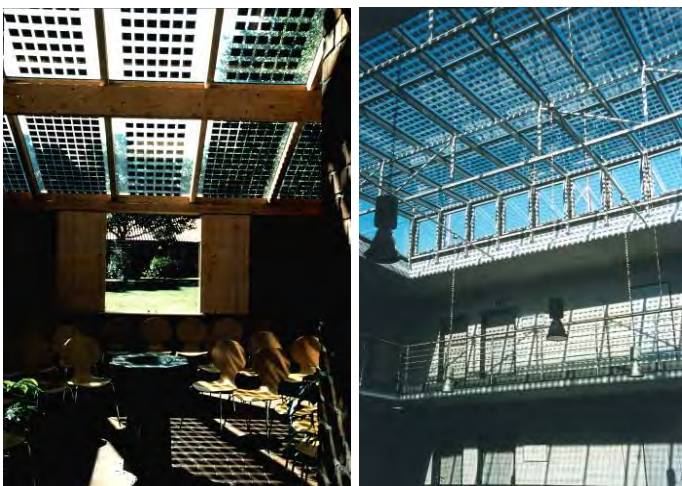
Fig. 17: Winter garden (left) and atrium glazing (right) in combination with semi-transparent photovoltaic roof elements (solarnova).
