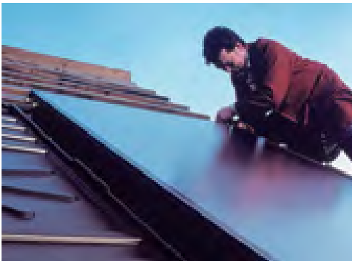
Fig. 24: Glazed solar thermal collectors on a flat roof (Energie Solaire, top) and integrated in a tilted roof (Buderus, Bosch Thermotechnik GmbH, bottom).
