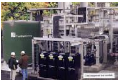
250-kW FUEL CELL UNIT at Yale University in Connecticut, U.S.A.
